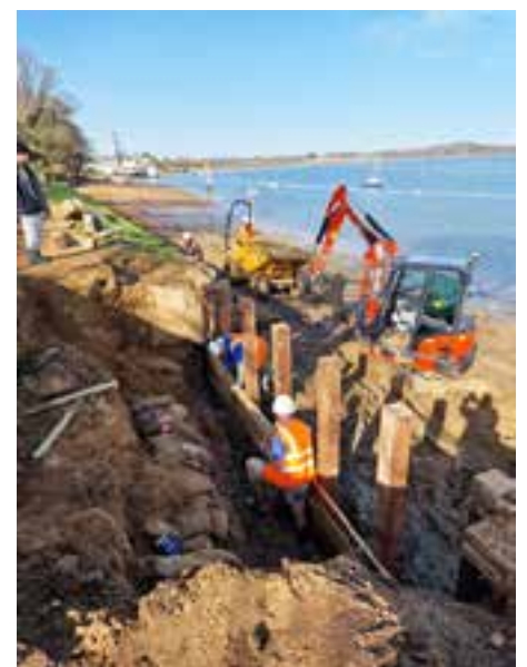
Estuary bank repairs at Waldringfield
