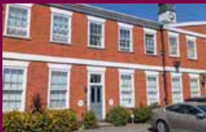
STATION ROAD, LEISTON
