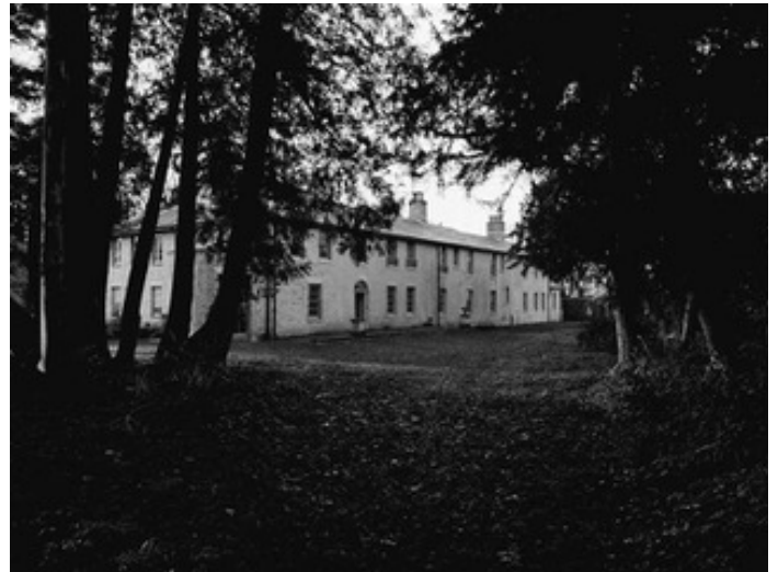
Great Ashfield House
